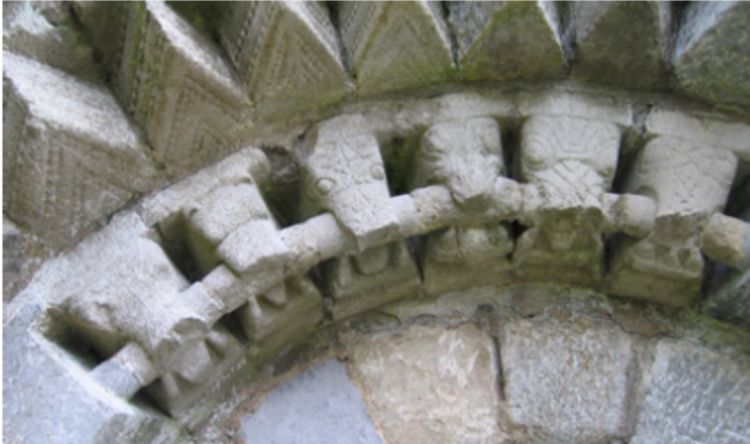
5. Detail of western portal, Nuns' Church (Photo courtesy of author)
